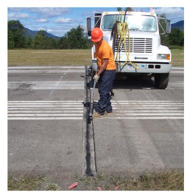
The Heat Lance is used to dry and prepare pavement cracks, potholes, and other distressed pavement surfaces for repair. It offers separate valves that control the mixture of fuel and compressed air at the point of combustion.
